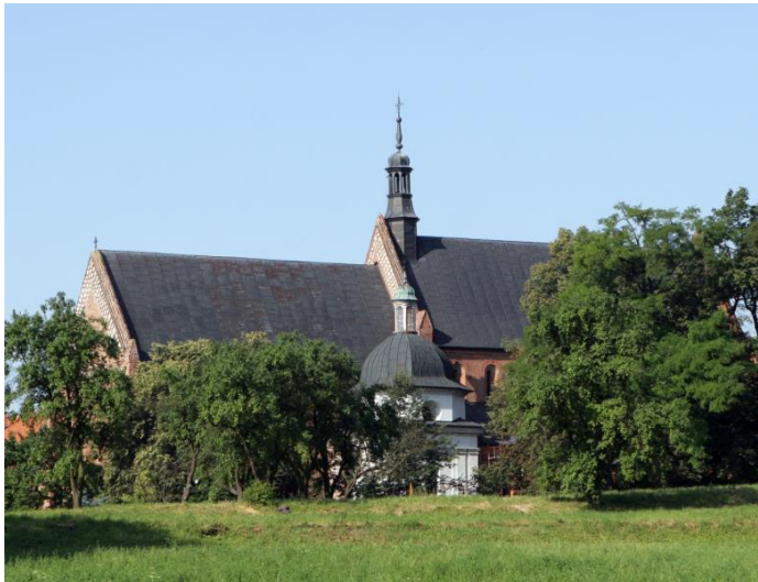
The Church of St. James in Sandomierz (view from the north)
